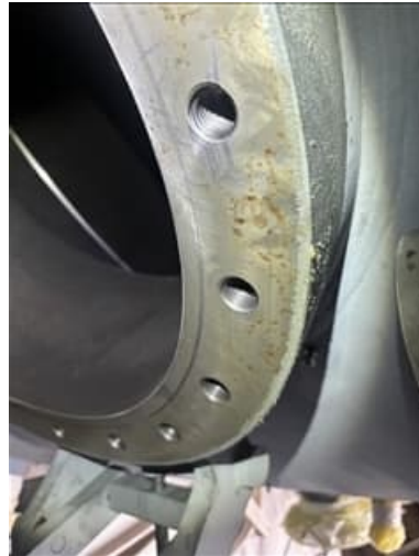
The lower outer manhole (3)
